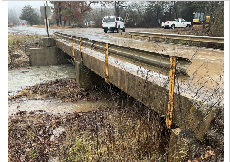
Typical bridge railing
