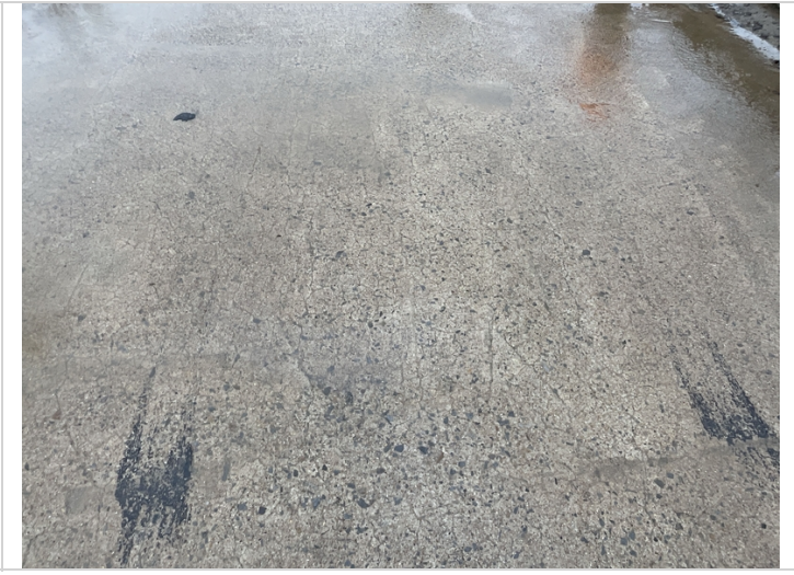
Typical map cracking through towering surface
