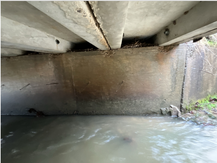
Bent 1 Units 1,2 3 spalling in bearing area
