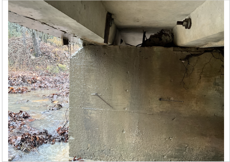
Bent 2 Spalling in top of pier wall
