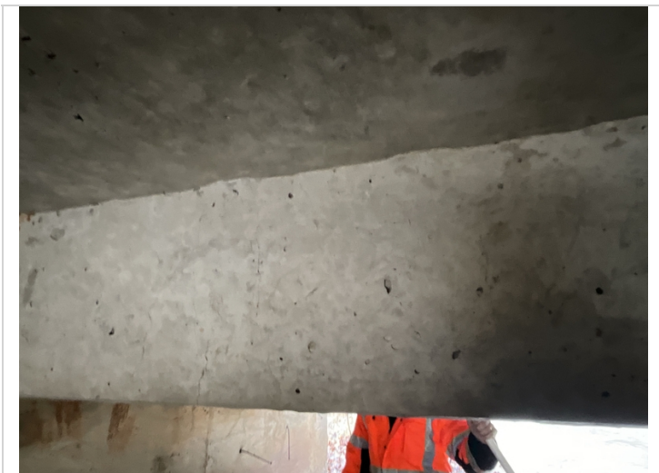
Typical hairline flexure cracking 1' centers
