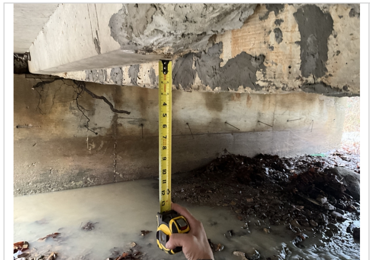
Span 1 Unit 2 has 2 1/2 " deflection no change
