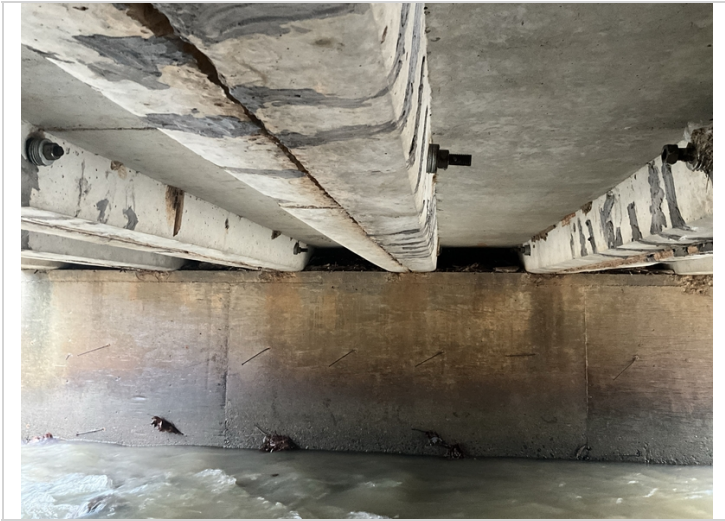
Span 1 Units have lose bolted connections
