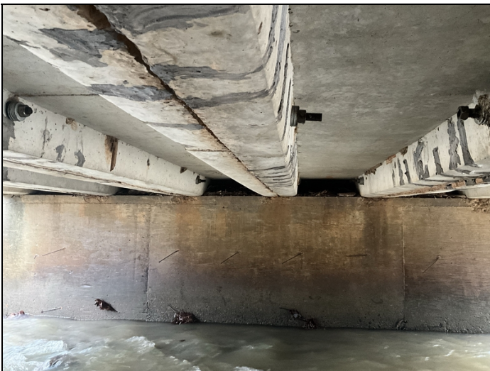
Span 1 Units have lose bolted connections
