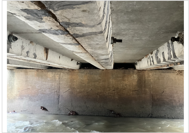
Span 1 Units have lose bolted connections
